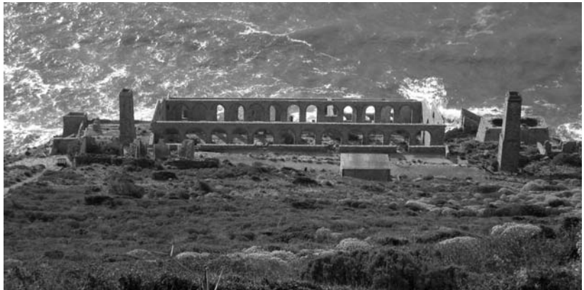
The Lamarmora washing plant (1897), at Nebida, south western Sardinia. Photo: David Worth
